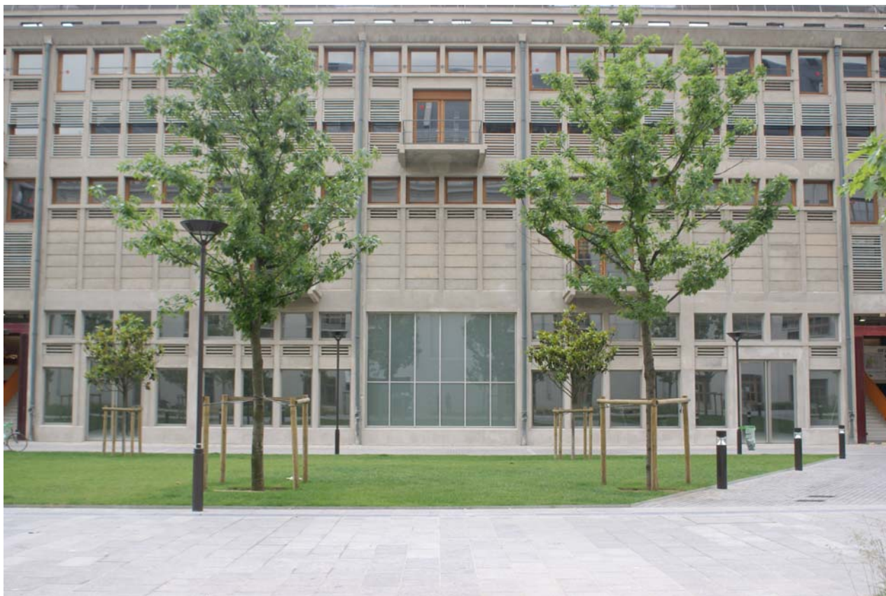
View of the façade of Bétonsalon
